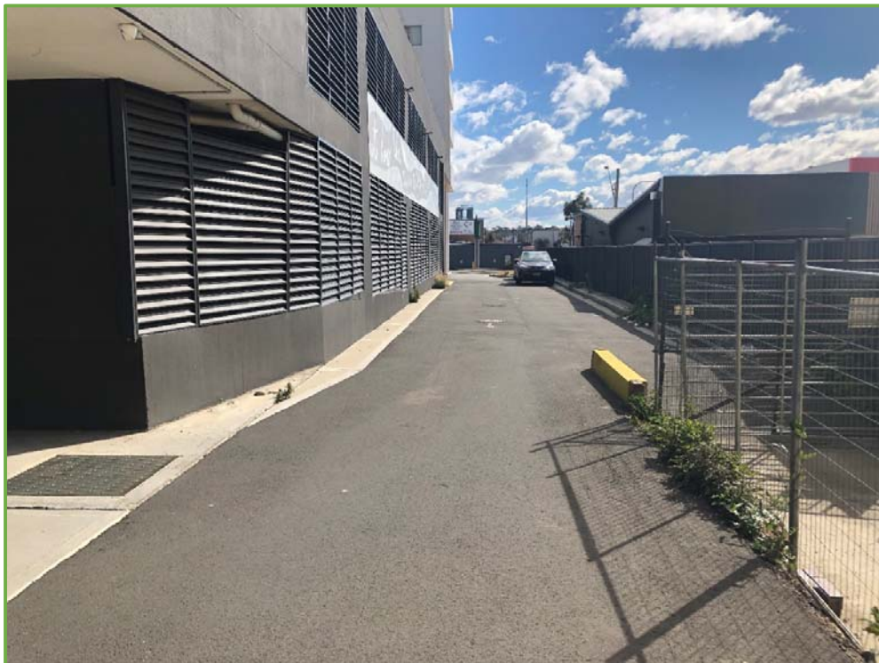
View looking north-west from unnamed laneway towards Bold Street
